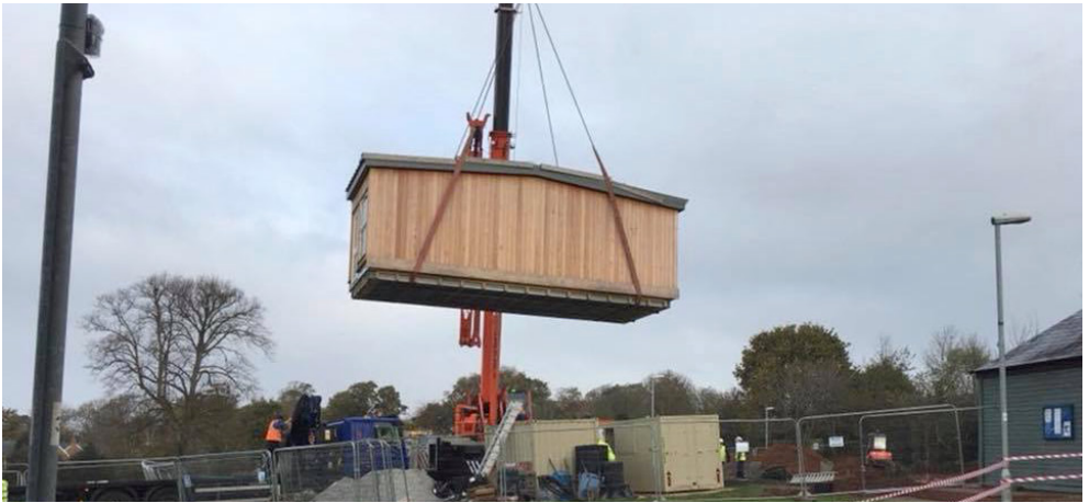
A SECTION OF THE NEW PRE SCHOOL BEING CRANED IN
